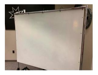
5. Hang the top of the boards to the top of the Z Rack using zip ties. Only tighten the zip ties once all the ties are attached and the holes are properly aligned.
