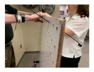
4. Place the peg board and painted plastic panel back-to-back and thread zip ties through both boards.
